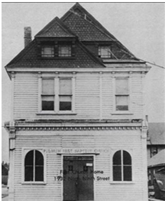
1932 North 9 th Street September 15, 1952
